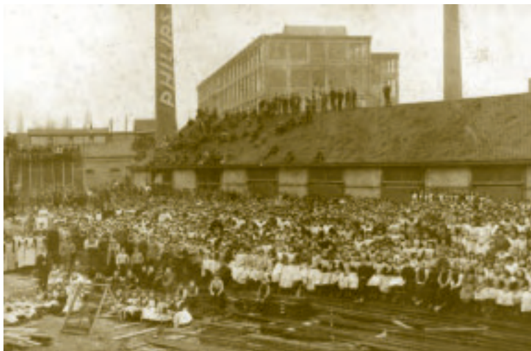
The Philips transformation: from its beginnings - here a plant in Eindhoven 100 years ago - as a lamp manufacturer ...
