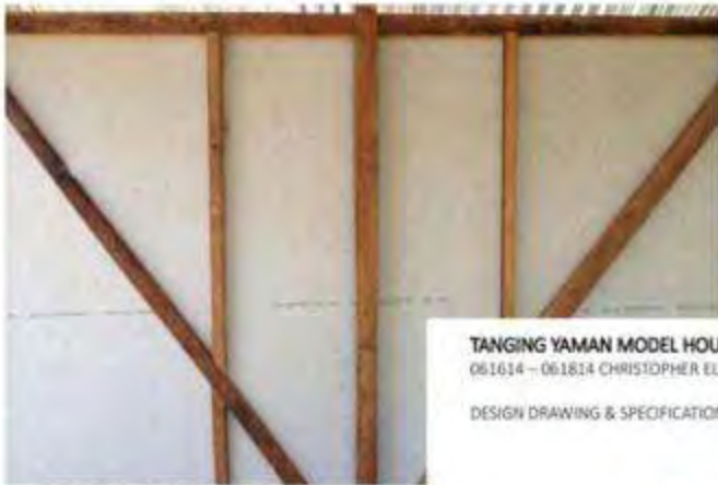
Interior view of hardiflex walling showing the wood member
